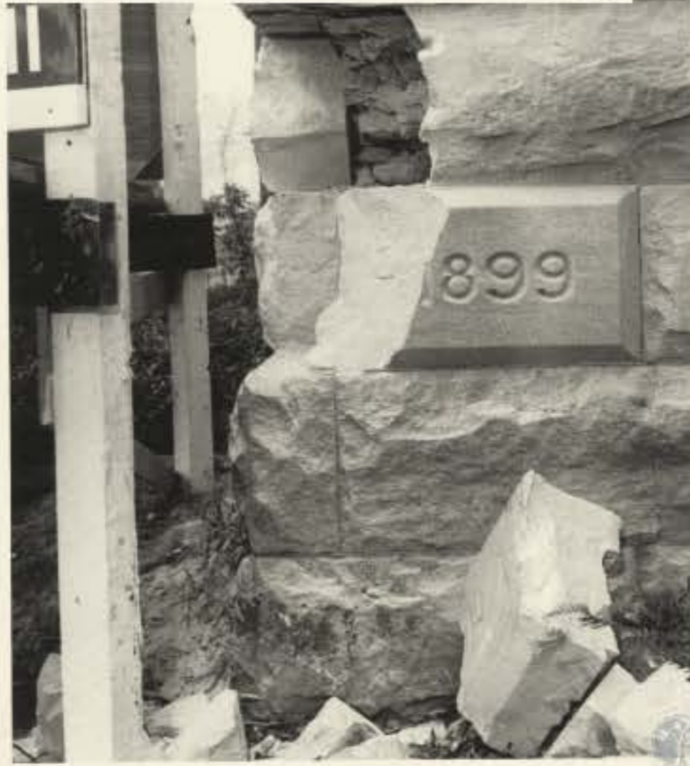
Cornerstone during 1970 demolition.
