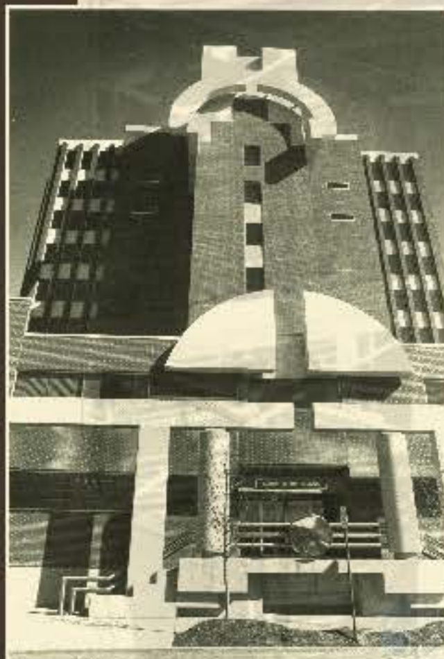
View from Scott Boulevard.
